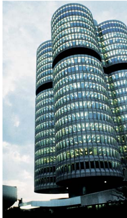
Fig. 1. Following its restoration, the BMW Tower is a beacon of energy efficiency and ergonomically designed lighting solutions
